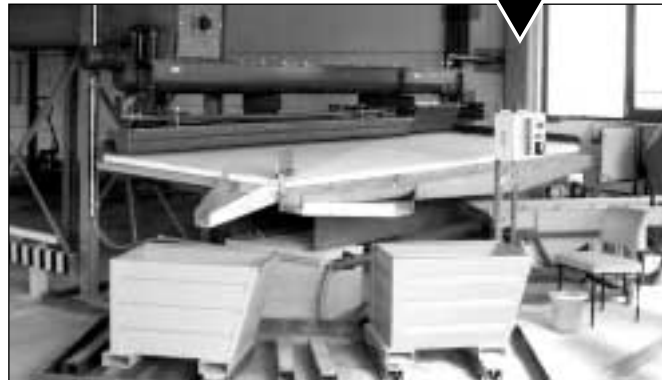
Wet table installation
